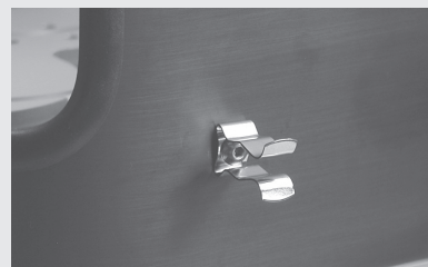
Figure 4.13 The grounding clip
